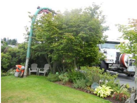
Figure 5-5. Excavating for Vac-A-Tee.
