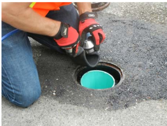
Figure 5-9. Folding Plug in Half.
