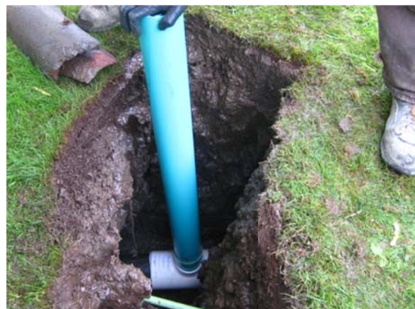
Figure 5-6. Attaching the Vac-A-Tee.
