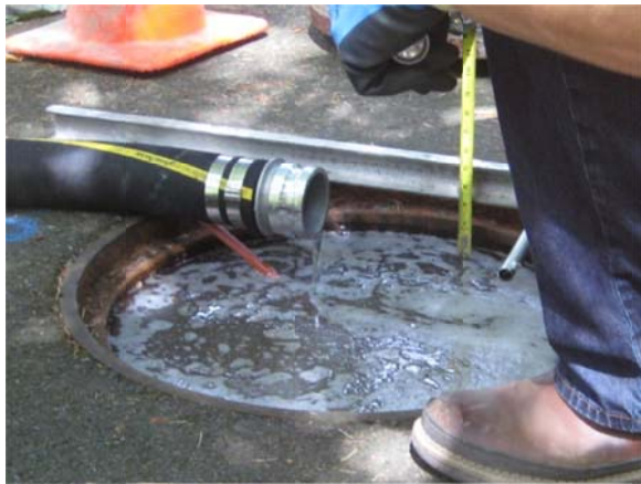
Figure 5-11. Filling and Measuring S1.
