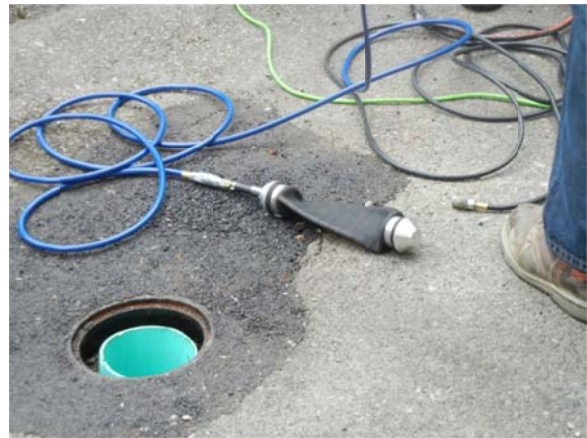
Figure 5-8. Deflated Plug Prior to Insertion.
