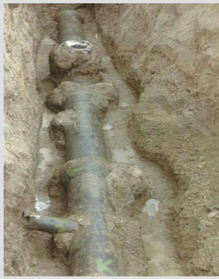
Excavated trench after sealing the pipe
